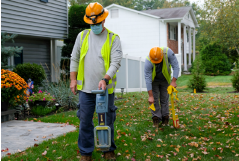
Two O&R damage prevention technicians team up to locate and mark out underground O&R gas and electric facilities at a home in Nanuet. In the foreground James Mischuk uses a radio detection receiver to locate O&R underground gas facilities while J.D. Gallo follows to mark the locations with paint and flags. This procedure warns excavators to avoid digging near the facilities.
